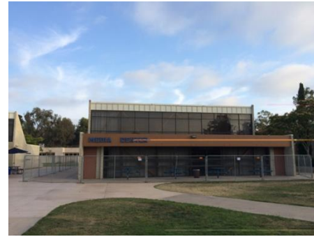
DNO Student Circulation, Media Center & Technology Infrastructure
