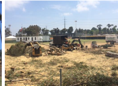
TPHS Weight Room, Fire Road, Chemistry Classroom Bldg.
