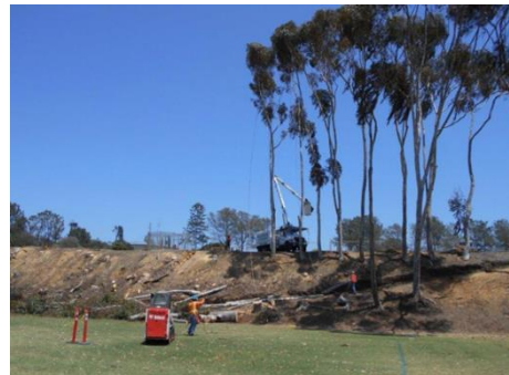
OCMS Ramp, Art, C-Smart Improvements
